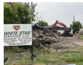
3115 McArdle Road Demolition
